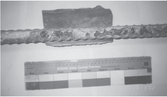
Figure 21. Localized corrosion in exhumed soil nail
